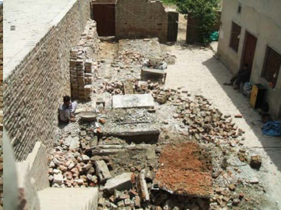
Opening the court yard for construction.
