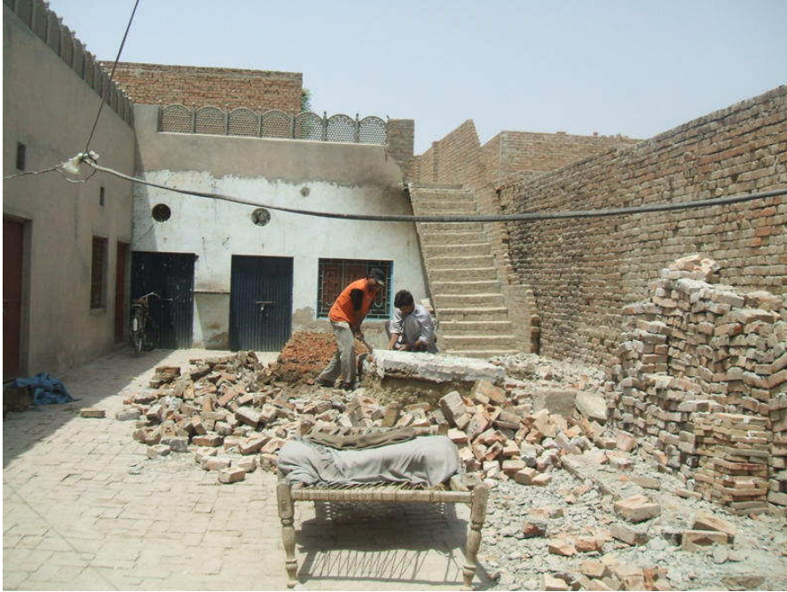
Preparing for new construction
