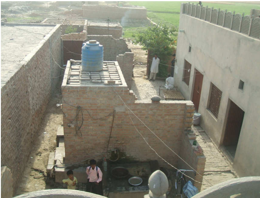
Inside courtyard before demolition
